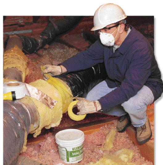
calibrated mechanical equipment to measure the amount of airflow that is lost through the duct system when it is pressurized to its normal operating pressure. While some joints or seams may have only small leaks, other sections may be completely disconnected. Duct testing can indicate the relative leakiness of the ducts and help determine if the duct system should be sealed, repaired or renovated.
